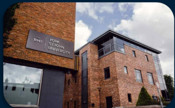
Figure 32: The Centre for Applied Innovation at York St John University
